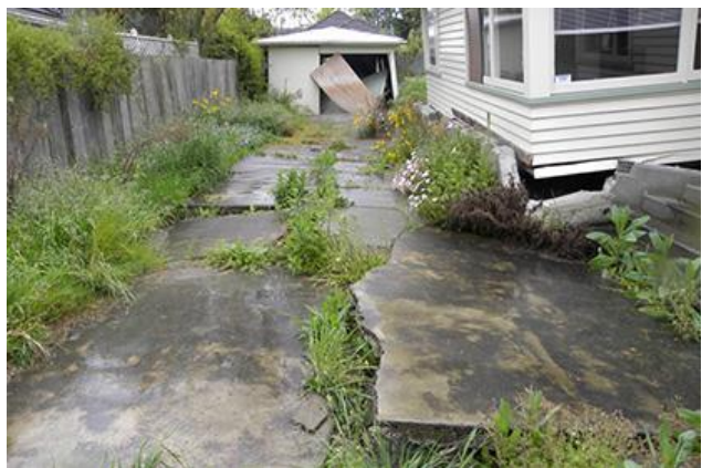
Fig 5.1.2 (b) Effect of soil liquefaction
